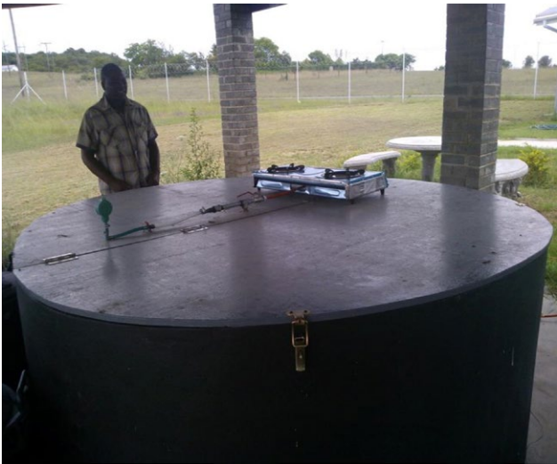
Figure 5: Sawdust insulated biogas digester for energy generation
